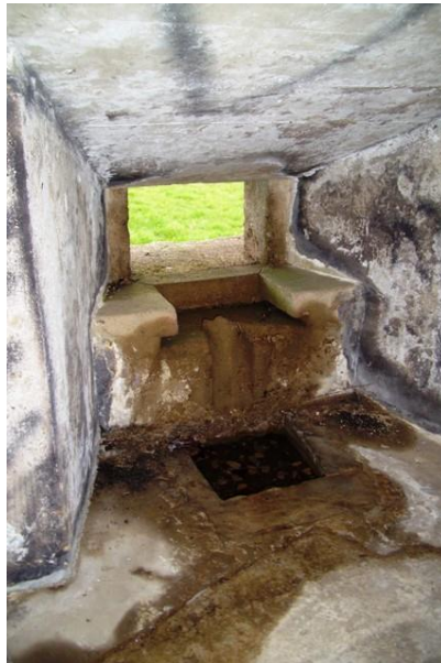
Loophole for the Bren LMG, note well for front tripod leg.
