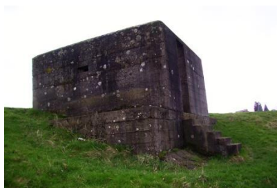
View of pillboxes substantial foundations and entrance steps.
