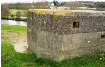
Close up of chamfered corner and fume vent.
