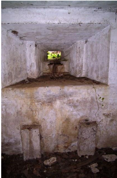
Bren Gun LMG loophole with tripod leg supports.
