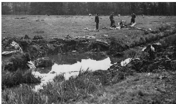
Example of crash site showing crater and furrow dug by a crashing aircraft 38
