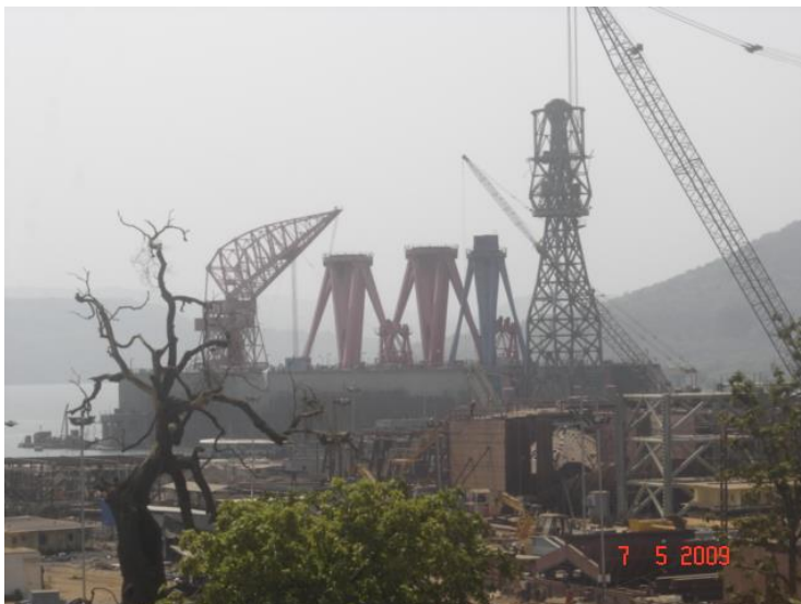
Floating dock fast in temporary berth, Bharati Shipyard
