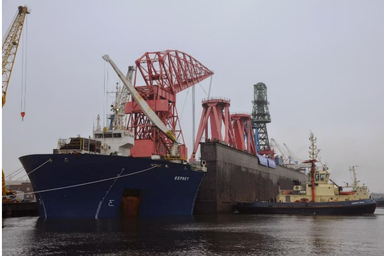
In position over the cargo deck.
