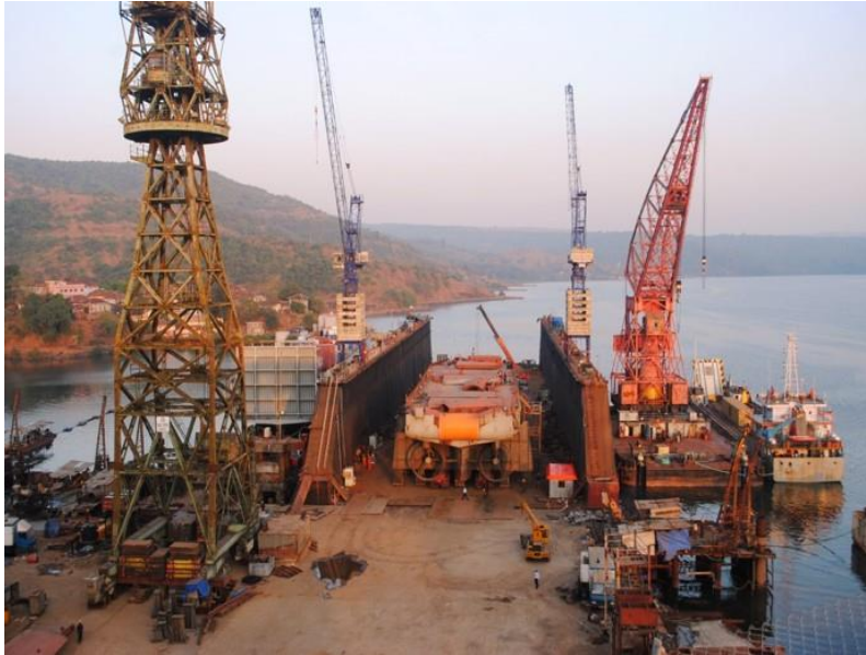
Floating dock and cranes in operation subsequently
