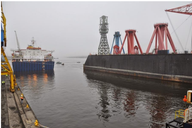
Osprey cargo deck submerged. Floating dock positioned ready for the floatover.
