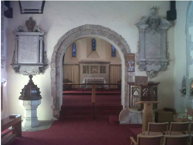
Re-used Roman monumental tufa entrance arch, All Saints Church, West Farleigh author, 11 June 2011.
